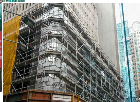
Alterations & Additions Works
