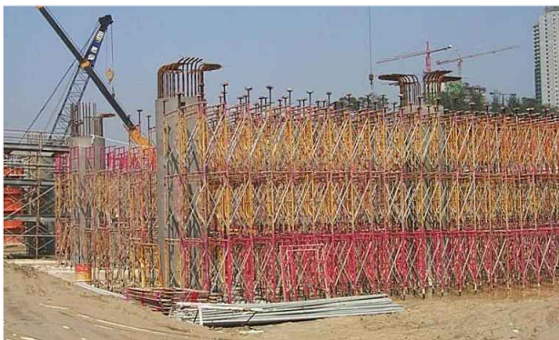
Toyo Scaffold Support for Concrete Slab
