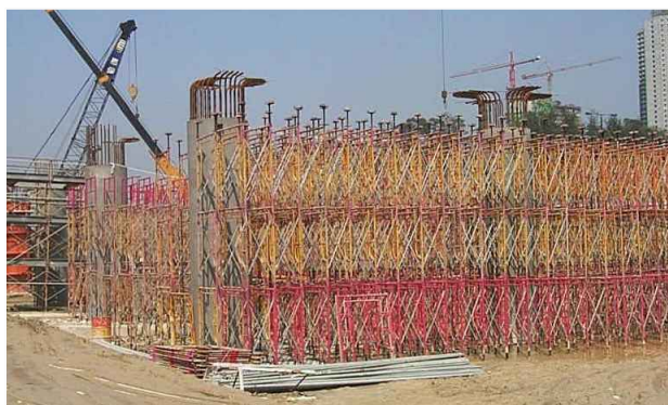
Toyo Scaffold Support for Concrete Slab (under-construction)
