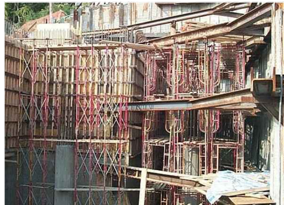
Toyo Scaffold System for Falsework
