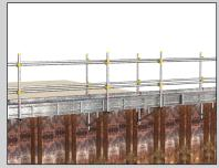
Step B3. Repeat above steps and install corresponding scaffold accessories to complete an edged-protected walkway on a sheet pile wall.
